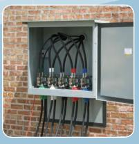
Berthold Electric Company's Generator Connection Cabinet provides a quick and convenient station to connect a portable generator to a facility's main service entrance equipment. Whether during a long-term utility outage or planned facility maintenance, our cabinet will help you easily establish a connection to back-up power when time is of the utmost importance.
